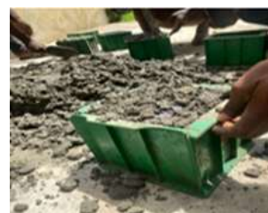
Figure 4: Mixing and casting of concrete
