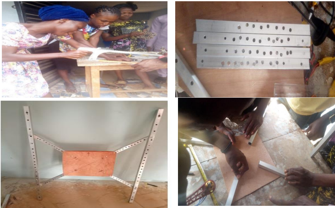
Figure 3: Drone Frame Construction
